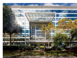
DIAGONAL 640 Barcelone (Spain)
